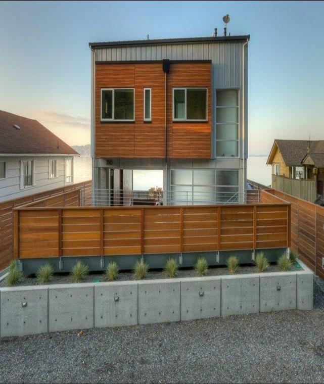
The Tsunami House, on the northern end of Washington's Camano Island, is designed to withstand the impact of powerful wave walls with heights of up to eight feet and speed up to 136 kilometres
